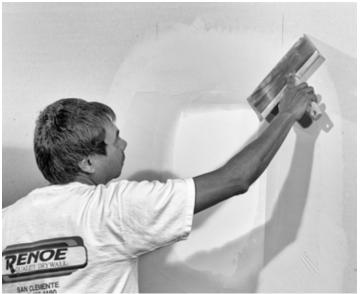
9. Build layers of compound as needed to obtain a flat surface. 11. Allow first coat to fully cure or harden.
