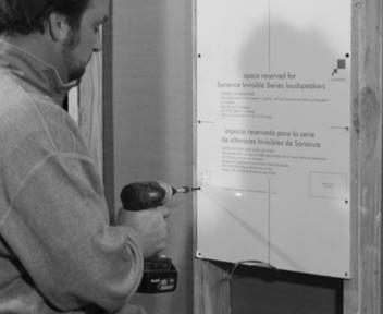
5. After all drywall is hung, begin speaker installation by removing space saver.
