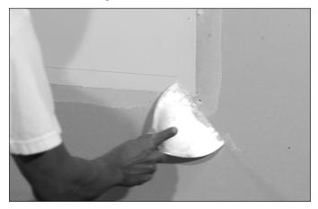
3. Allow hot mud to set slightly before applying mesh tape.
