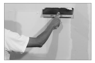
12. Detail the compound to minimize tool marks.
