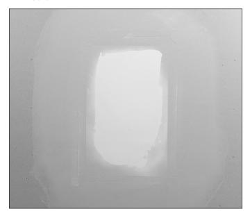
IMPORTANT: If a perfectly flat finish is achieved at this point, you may opt to proceed to the priming and painting phase. This is what we refer to as a "Finish Up To" installation. In this case, we recommend multiple layers of paint to achieve a shadow-less, even blending of color.
