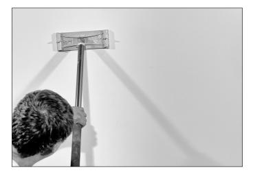
16. Validate the finish thickness using the Sonance DISC system and DG-1 depth gauge (SKU 93491).
