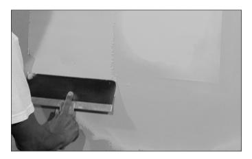
11. Compound buildup on the active surface of the speaker should not exceed 1/16" (1.5mm).
