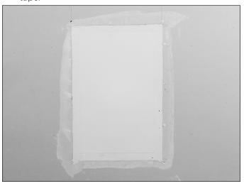
4. Place mesh tape over the drywall seams. Overlap tape slightly.
