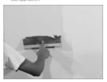
15. After final coat is applied and has dried, use a manual pole sander or block sander on entire wall (do not use a power sander as this could damage the surface of the speaker). Be careful not to sand down into the surface of the speaker. This could damage the paper which makes perfect blending very difficult to achieve. Wall surface should show no signs of a speaker.
