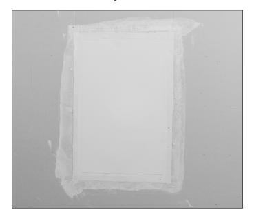
7. Once hot mud has fully cured, cover joints with slow-setting compound.
